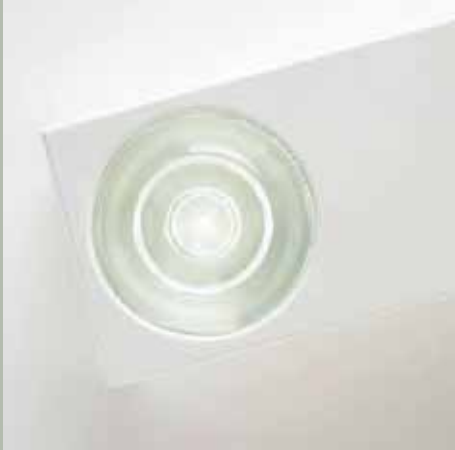
K7 permanente anti paniekverlichting - webref. SK7008A2
