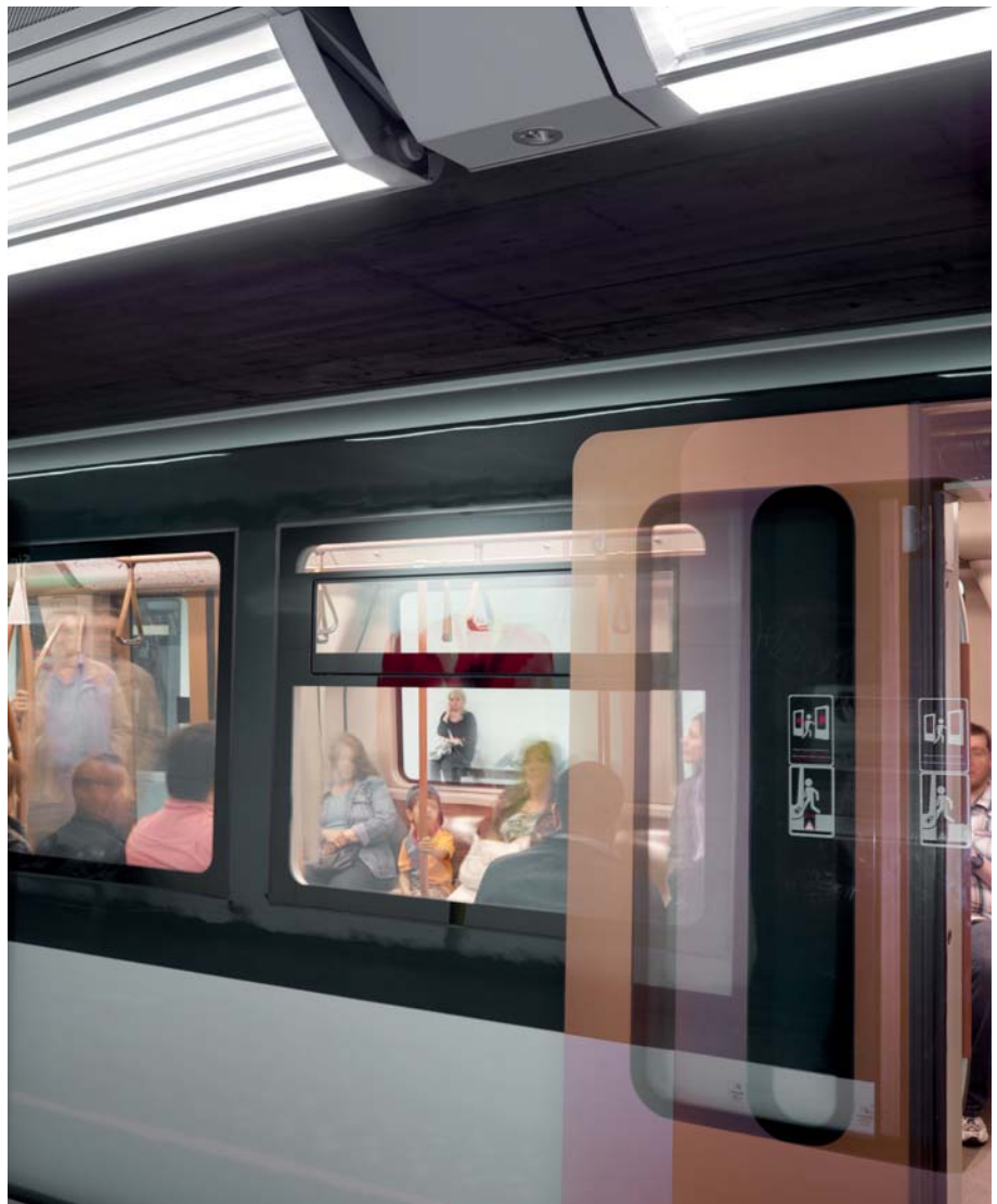
STIB-MIVB, BRUSSELS - BELGIUM integration of emergency lighting webref. SK9014D4
