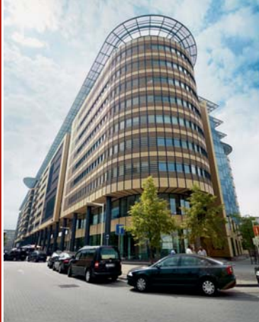
Regie der gebouwen (Victor Horta building), Brussels – Belgium – webref. SA021AA2
