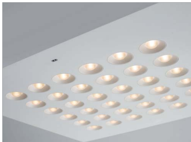
U7 with daylight dependent light control (ELS)
