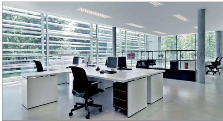
U7 luminaires in an office environment have a maintenance factor of 87% after 50,000 burning hours (see table).
