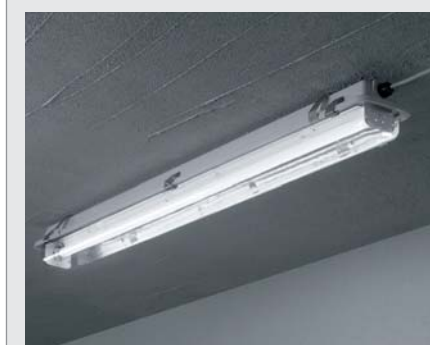
Fig. 38: While an E12/136HFW (with a 1 x 36W-fluorescent lamp) achieves a luminous flux of 3350 lm, and an efficacy of 72 lm/W, the same device with LED-tube achieves, respectively, only 1340 lm and 61 lm/W. Also, the light distribution with a LED tube (right) is different than the one with fluorescent lamp (middle).
