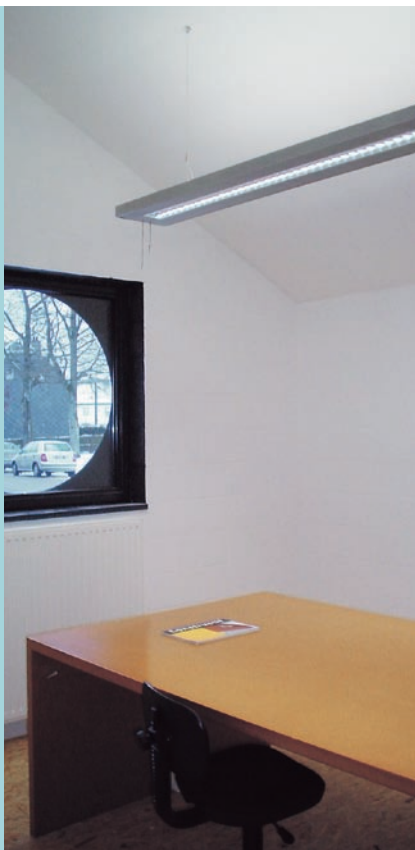
Suspended luminaires with connectable direct and indirect light for lighting small offices.
