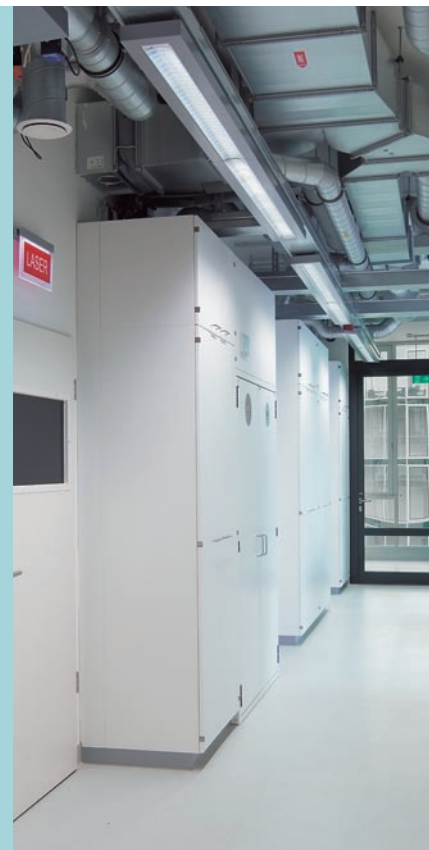
Enclosed luminaires with a transparent protected reflector.
