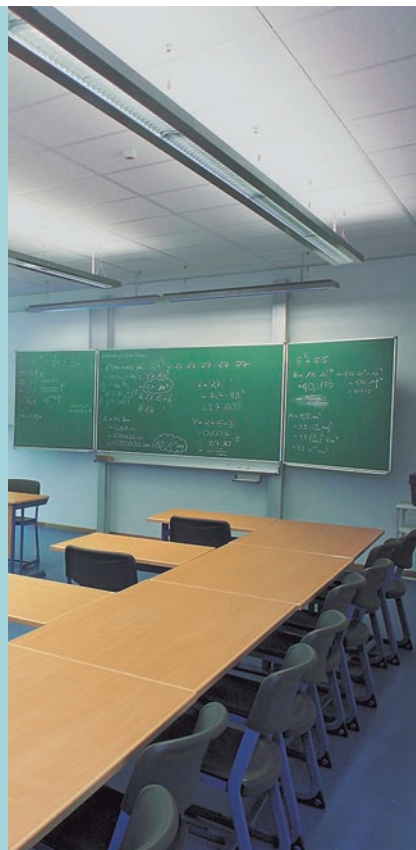
Wallwashers for illuminating vertical surfaces.
