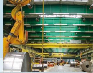
that as few as 204 [2 x 80W] luminaires (industrial E52 line luminaires) would do to achieve the intended 350 lux on the work floor. Quite a pleasant surprise in terms of the energy bill: 22 % better than the specifications. Compared to the old configuration, savings of no less than 46% were achieved. Furthermore Wälzholz had all luminaires fitted with daylight control to enhance energy savings.
