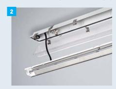
Screw down the new brackets and connect the LED module (by simply plugging in).
