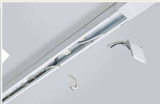
2. Remove end caps and connection
