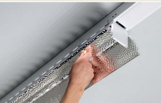
1. reflector demonteren
