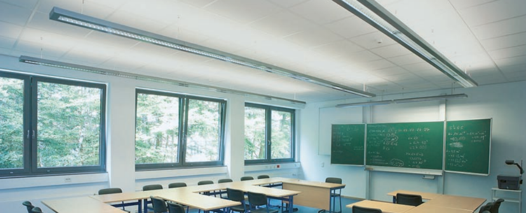
R4-luminaires integrated in a DALI-network ▶
