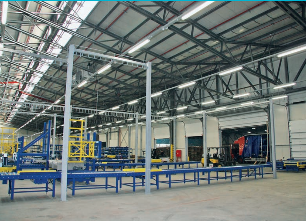
Crate washing facility: 440 individual E12/135 DALI luminaires
