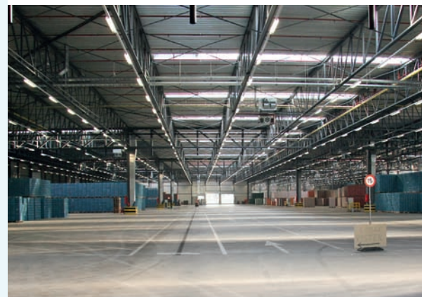
New hall with 1,000 E5200/280DALI luminaires on light lines
