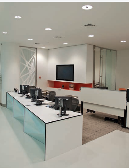
Efficient mix: the installation for Dubai Chamber included custom made fluorescent luminaires, D4 downlights with LEDs, and K9 emergency lighting with LEDs.
