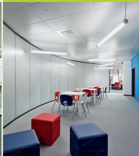
R8-pendelarmaturen in de coffee corners.
