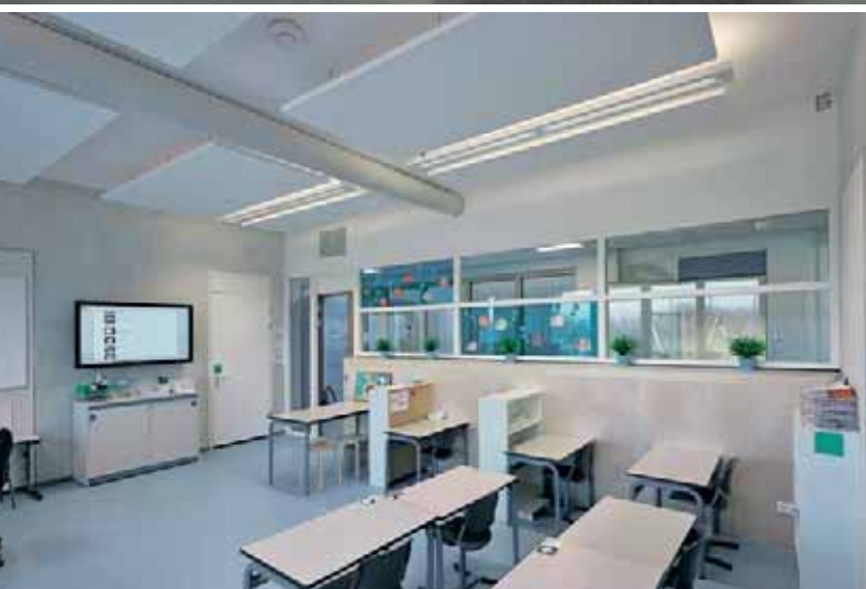
The energy-efficient suspended R4 luminaires with integrated uplight tie in perfectly with the acoustic ceilings.
