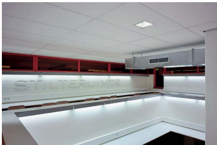
For grammar school Het Vlier in Deventer (the Netherlands), a light control system was designed based on five strategies. Thanks to a.o. presence detection and adaption to the task, 70% energy is saved per year.
